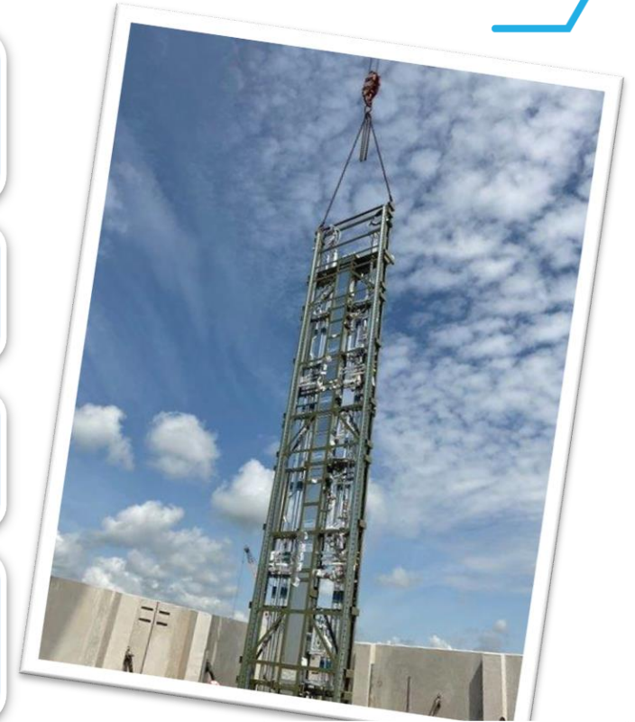
Modular riser being craned into position on site.
